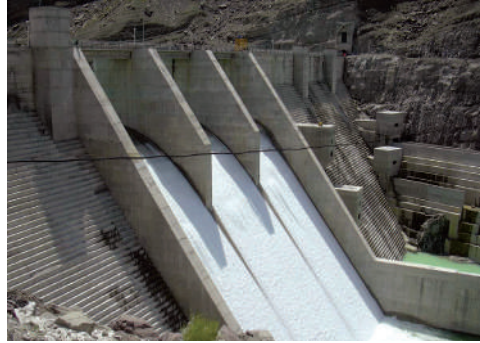
Climbing formwork system formed also stilling basin massive walls.
