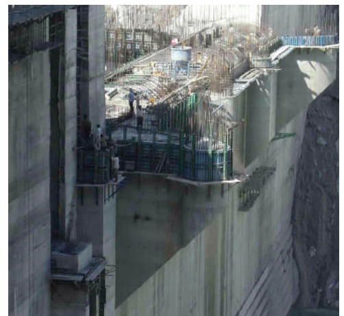
Safe working Platforms with modular Brackets.
