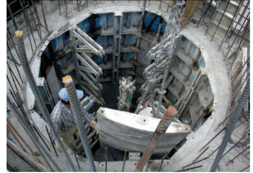
RCC shaft formwork is adapted to continuously concreting method.
