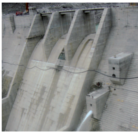
For the construction of the massive walls of spillway and irrigation outlets BFS solution were wall formwork systems and climbing Bracket.
