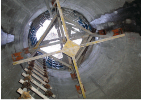
RCC shaft Formwork platform which means site personnel can always work safely.
