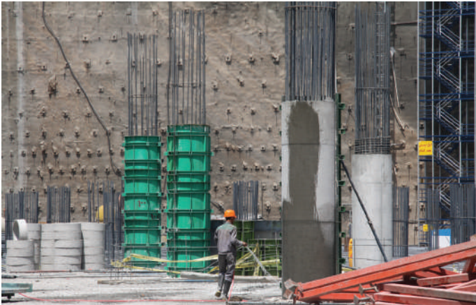
Circular steel column formwork can also use with the climbing system including brackets, adjusting prop,...
